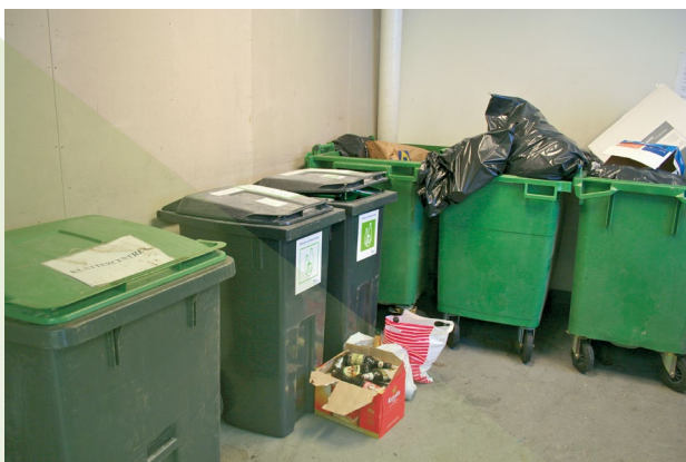
Garbage often cause odor problems in garbage rooms.
