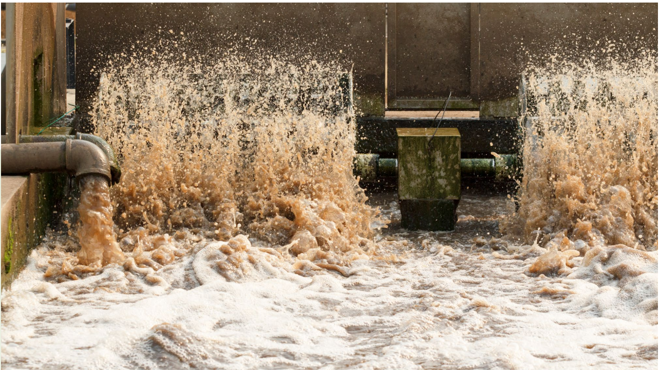
The groundwater that is collected to later be led to the stormwater drainage is often still and will eventually smell.
