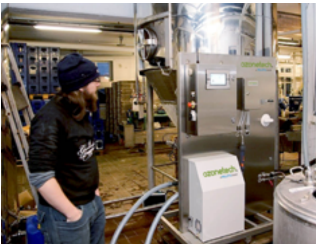
The Ozonotech RENA Vivo A-series system is connected to tanks and other process equipment during CIP sanitation. The brewmaster Johan Hansson is observing the system during operation.
