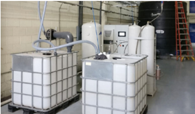
The complete solution designed by Mellifiq, including a complete Ozonotech ozone system with optimized ozone dissolution, control unit, oxygen system, cooling unit, reaction tank and foam collection.
