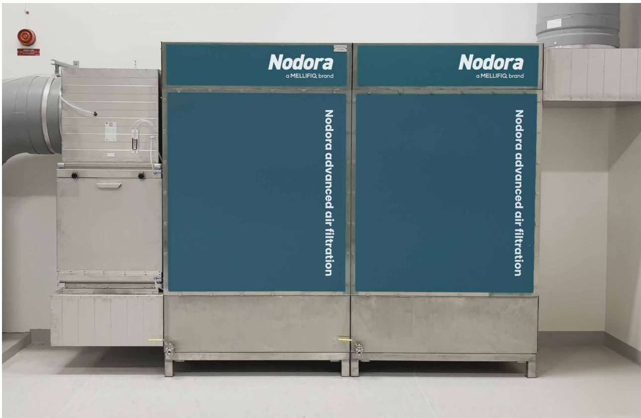
The first treatment step consists of two Nodora CAT modules tailored to remove high H 2 S concentrations.
