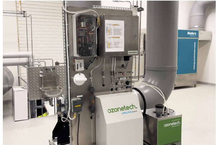
The RENA Pro systems produces the ozone necessary to eliminate the remaining odors after the Nodora CAT treatment.
