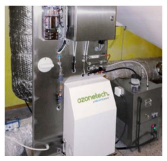
The Ozonetech RENA Pro is skid-mounted and installed close to the ventilation duct where the ozone is injected. The operation is automatic and the installation includes closed-loop cooling system, oxygen concentrator, ozone sensors and remote monitoring.
