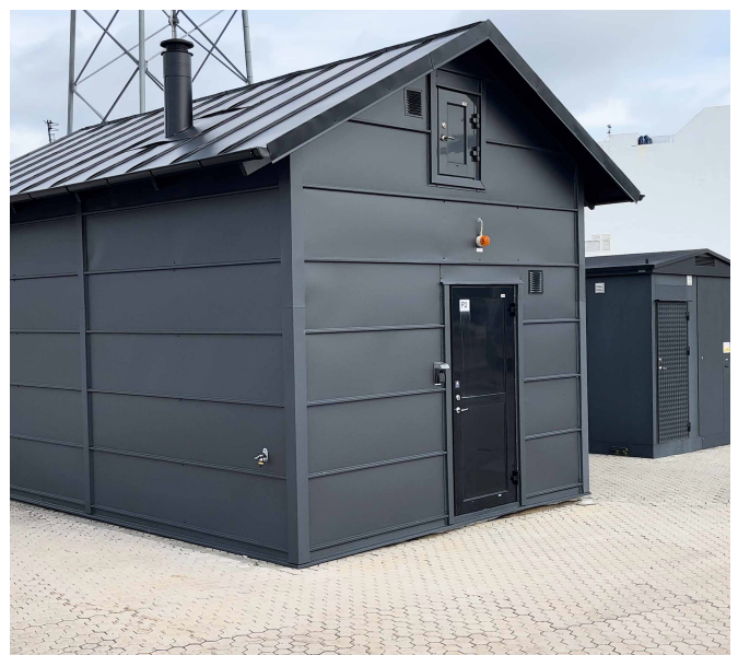
Outside view of the pumping station.
