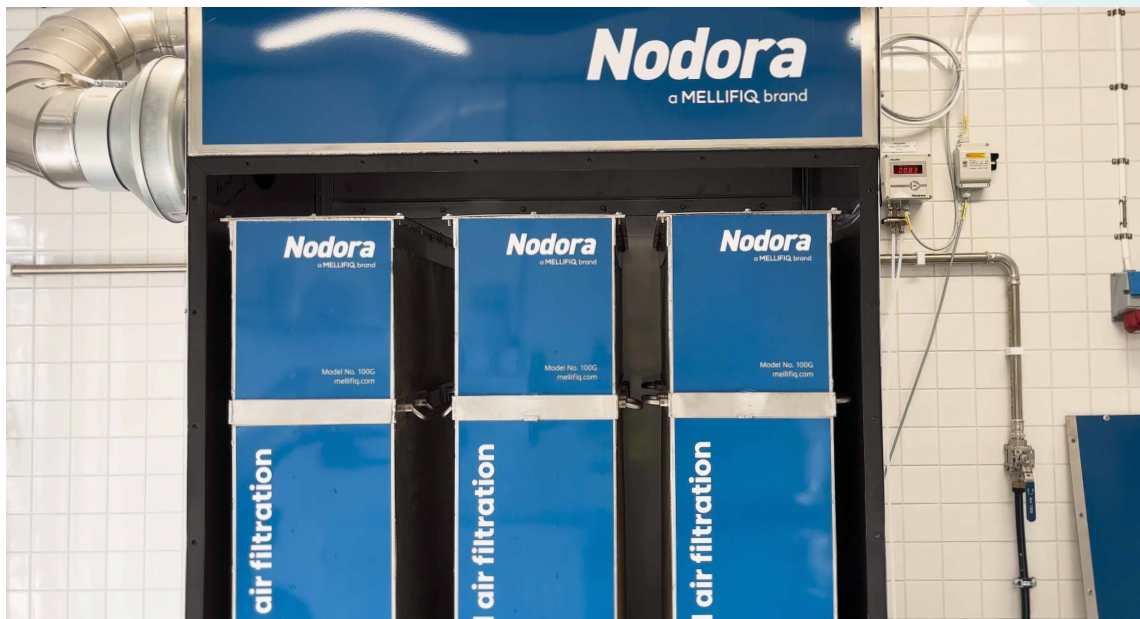
The three filter cassettes containing catalytic material, designed for easy maintenance.
